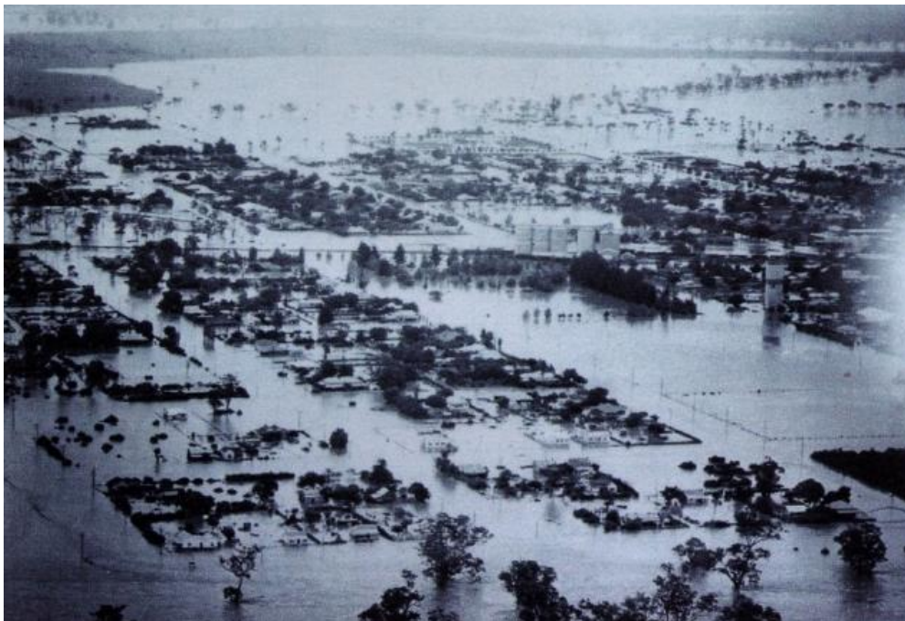
Aerial photograph taken looking south during the February 1955 flood, with the Macquarie River in the foreground.
